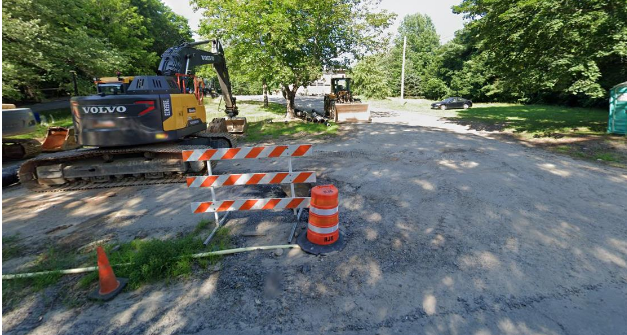
3 – View of the site’s existing southern entrance, facing the former John A. Andrews School building. This entrance will be improved to provide access into the proposed Senior-housing development.
