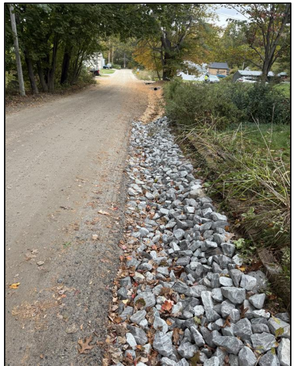
Figure 4. Proper ditching along Orchard Road.
