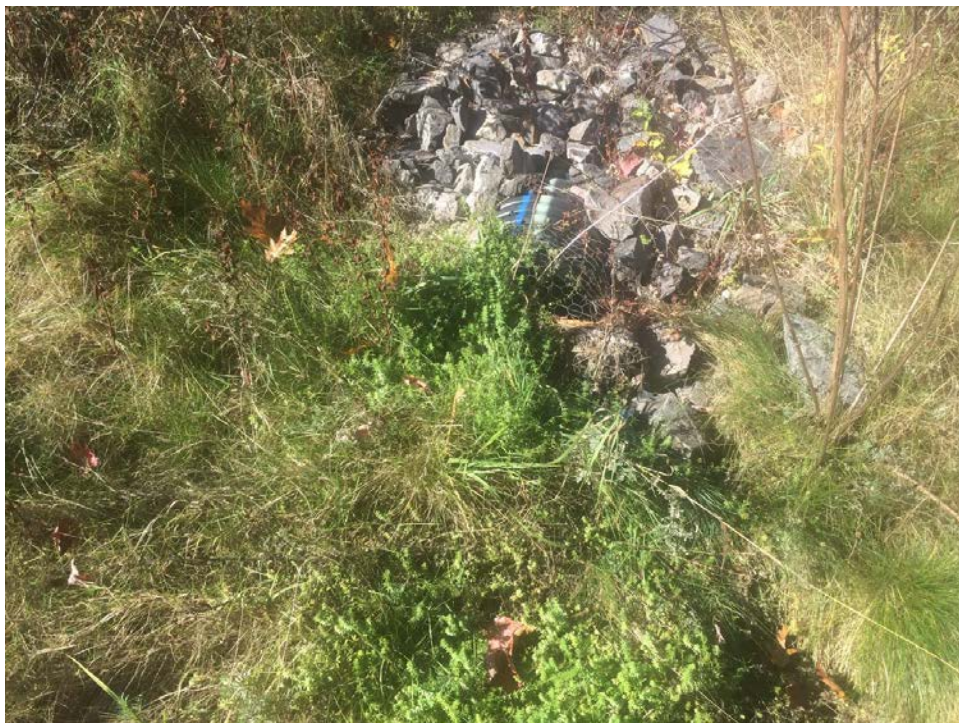
Photo 2 – CB33 outlet with vegetation overgrowing and obstructing the outlet flow.
