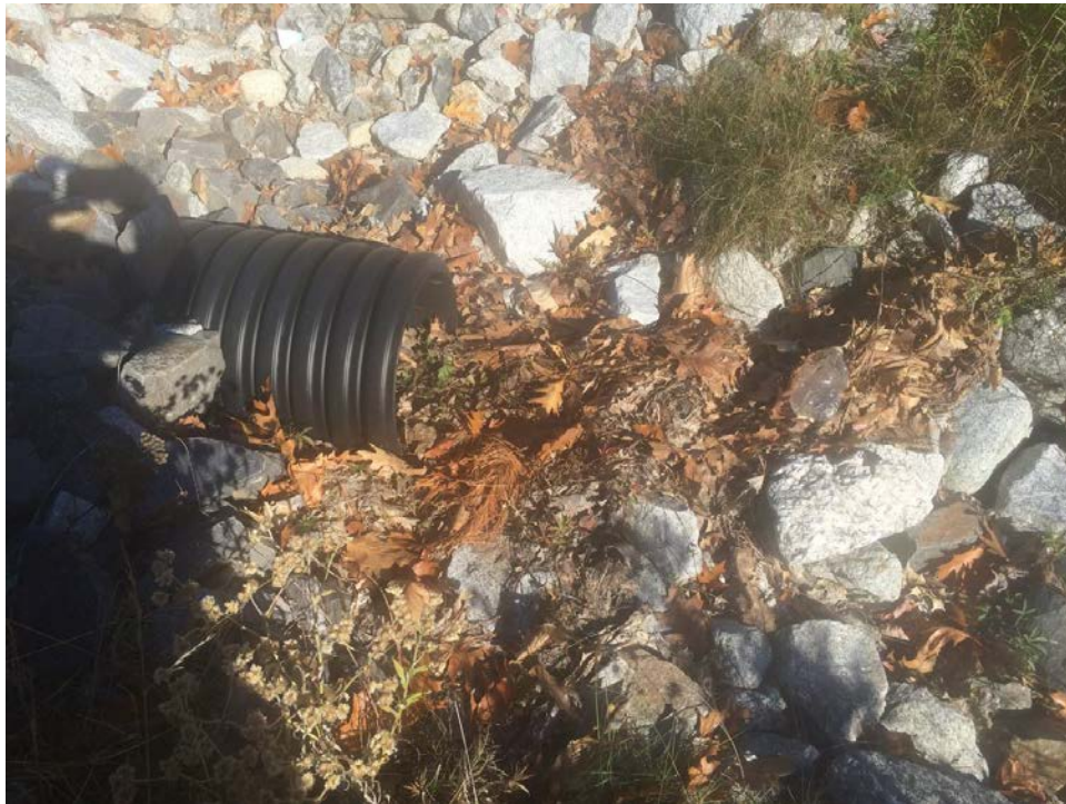
Photo 1 – CB34 outlet with leaves and sediment obstructing outlet flow.
