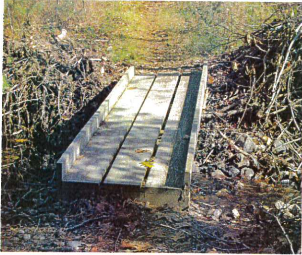
Figure 1 & 2 - Existing foot bridges
