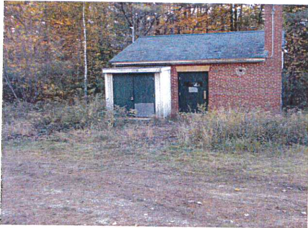
Figure 9 - 1 of 3 Utility Buildings on the property
