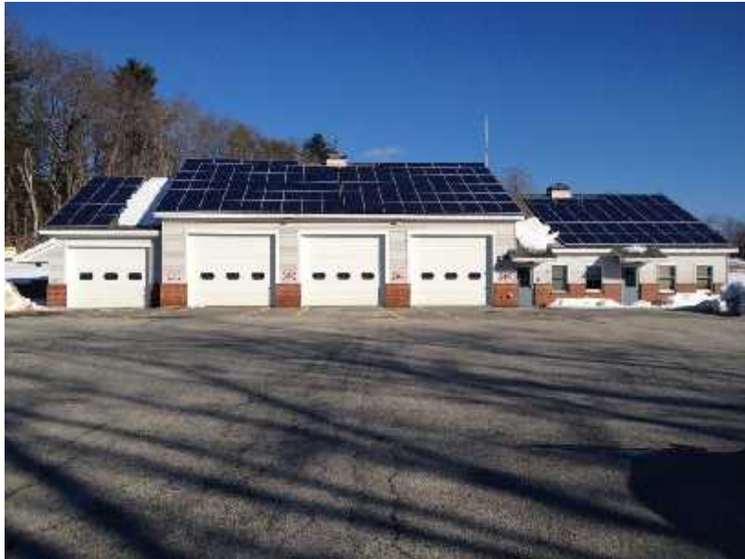
Figure 4 – East Windham Fire Station
