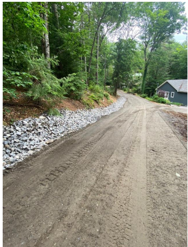
Figure 2. Reggraded road and new rip-rapped ditch
