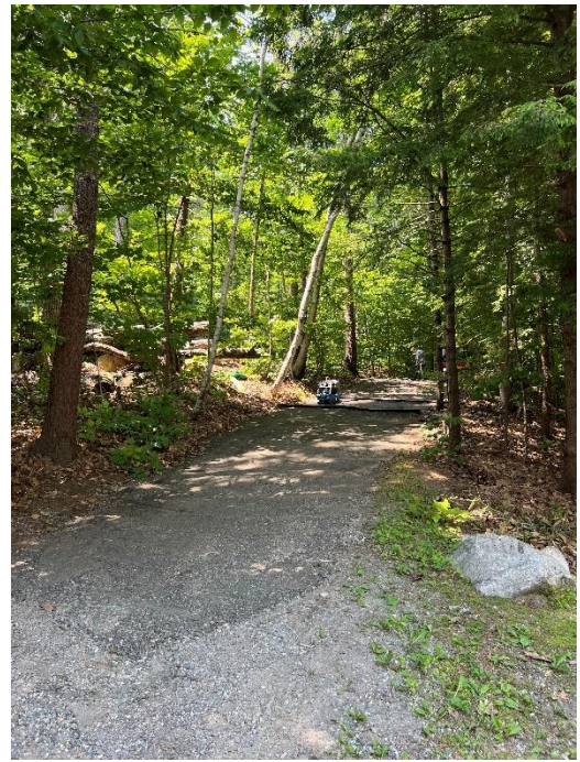
Figure 5. Regraded driveway and reset water bars
