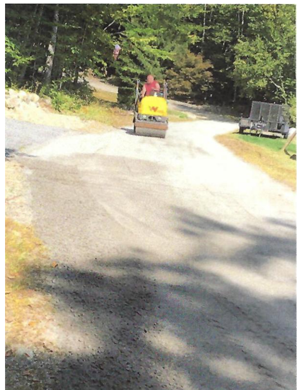
Figure 4. Proper compaction and crowing of road surface
