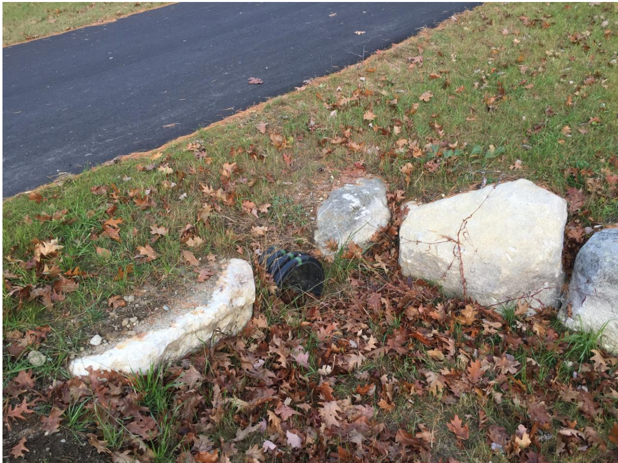
Photo 1 - Construct Riprap Aprons (#79 Harvest Hill Rd).
