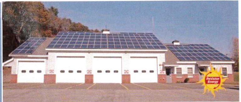
A 40 kW solar electric system installed on the roof of Windham's Fire Department by ReVision Energy
