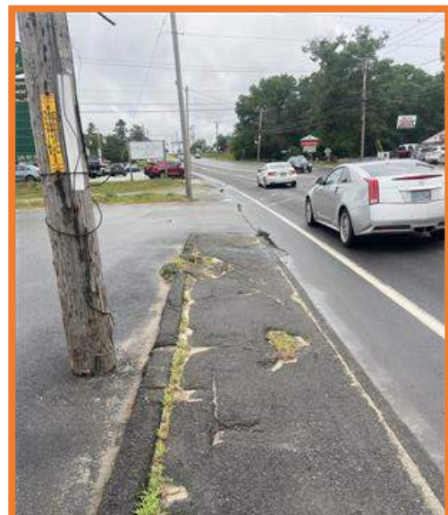
Example of sidewalk graded at ‘Severe’ (Roosevelt Trail)
