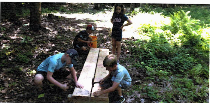
Standish Recreation Summer Camp Volunteers Building a Bridge.
