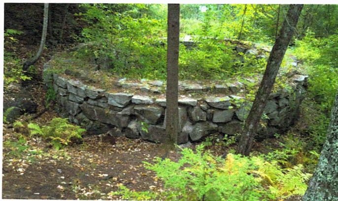
Gambo Preserve Mill Structure.
