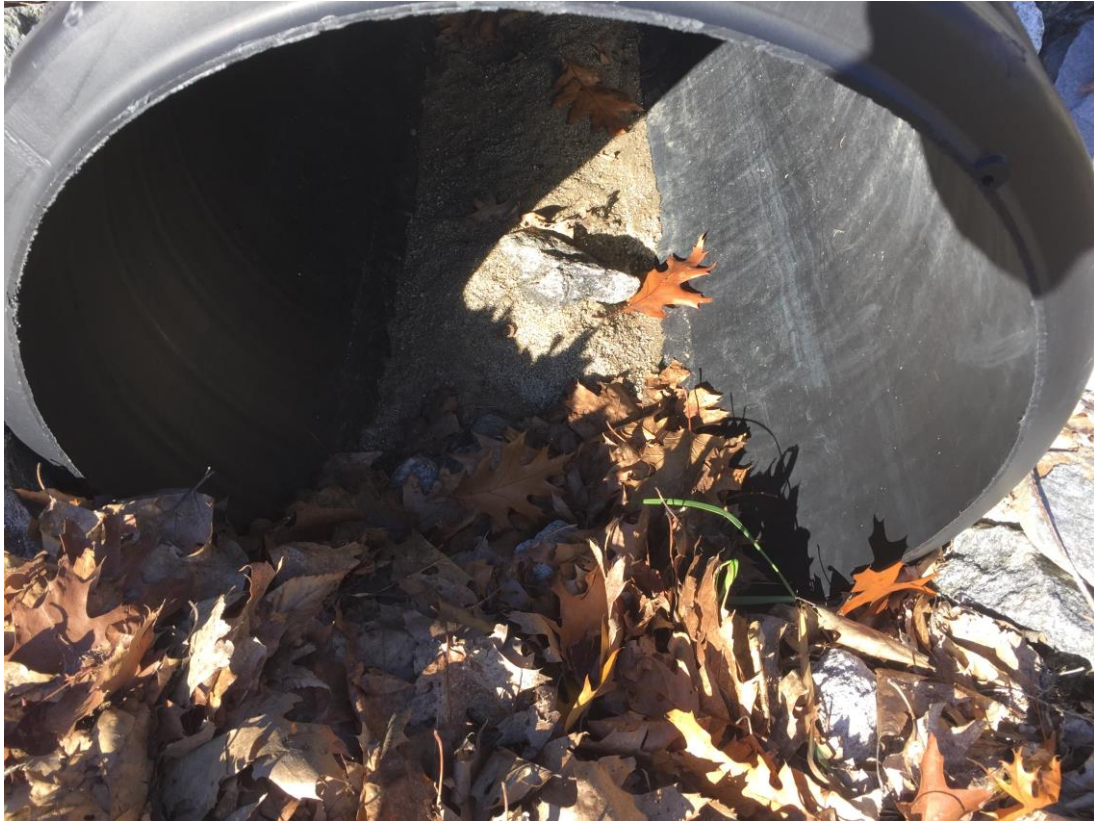
Photo #1 – Sediment Buildup in Driveway Culvert (Sta. 17+50, LT).
