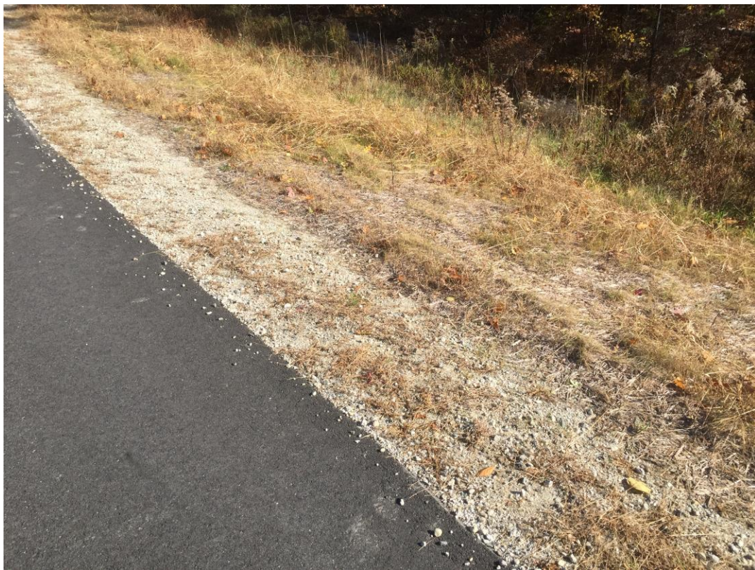
Photo #2 – Gravel Shoulder on Thrush Terrace (Sta. 12+00, LT).
