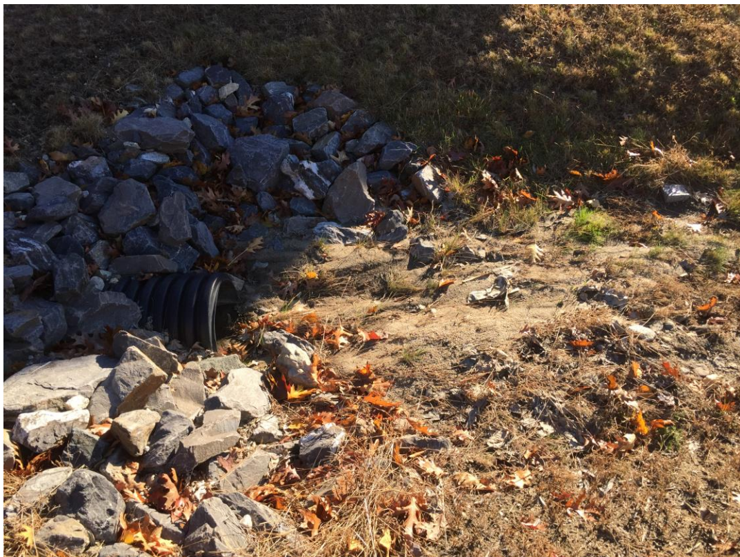
Photo #4 – Sediment Buildup at Driveway Culvert #47 Harvest Hill Rd (Sta. 26+00, RT).
