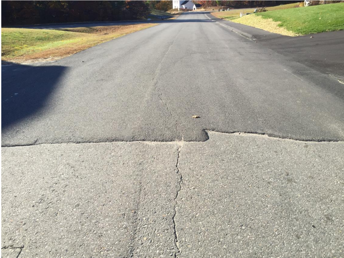
Photo #5 – Longitudinal Crack on Harvest Hill Rd (Sta. 26+50).
