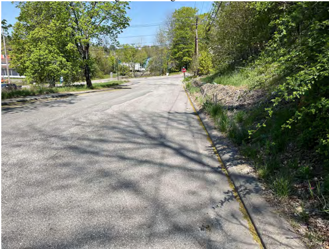
Photo 2 – Looking North on High Street from New Entrance
