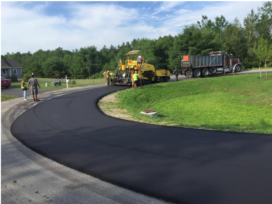
Photo 1 – Surface Paving Cul-de-Sac.
