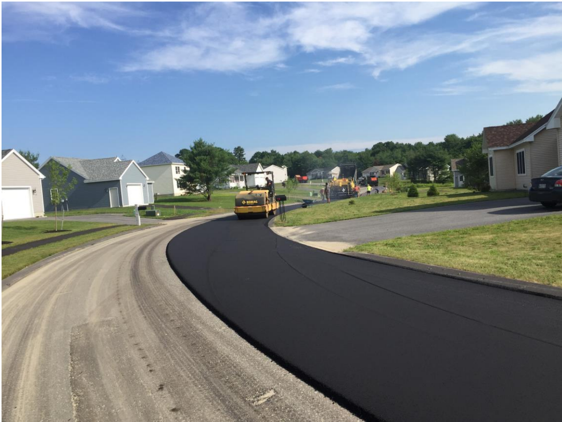
Photo 2 – Compacting Paving (Sta. 13+00).
