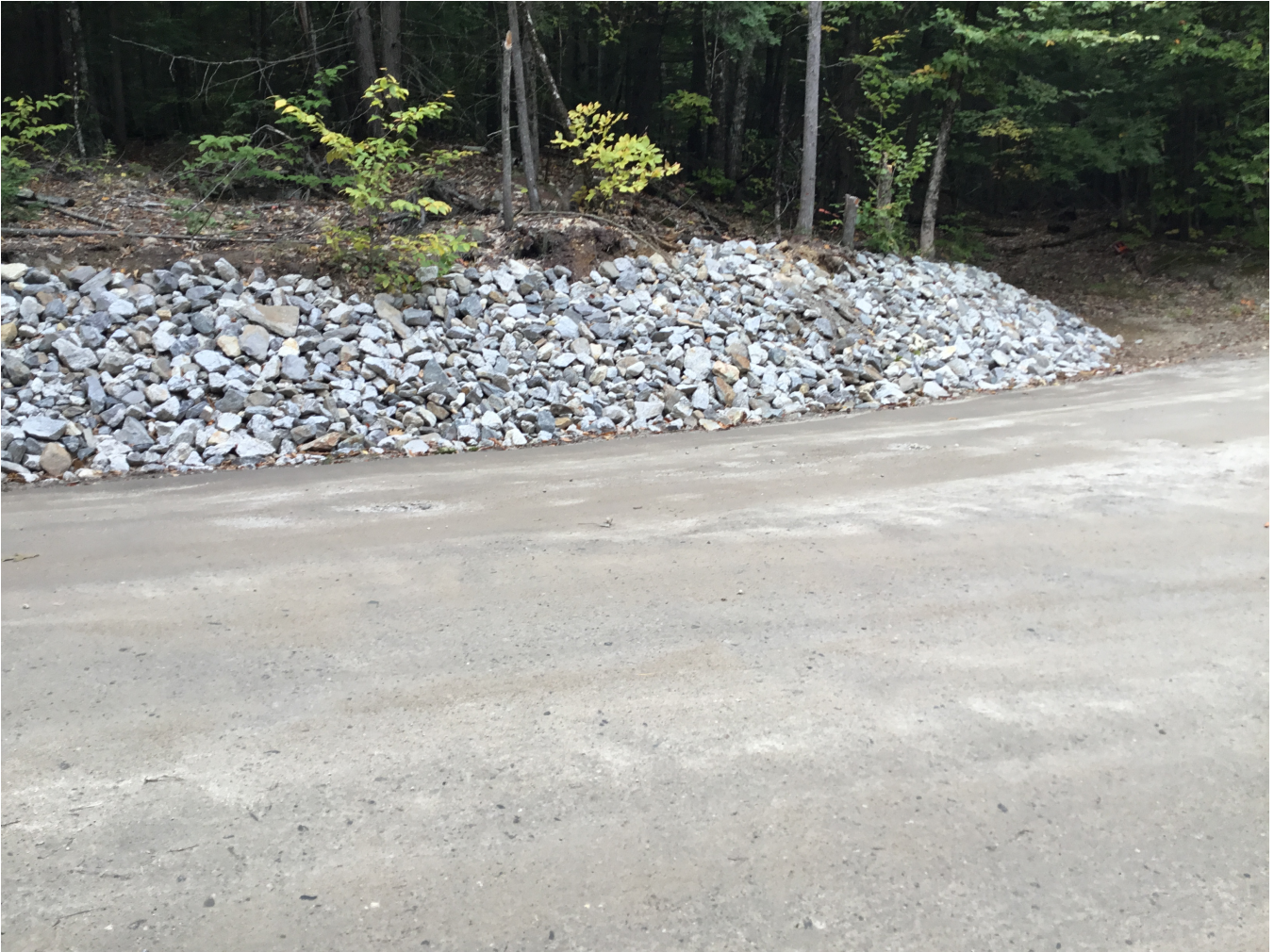
Stone rip wrap along ditch at gully erosion Site 5-2
