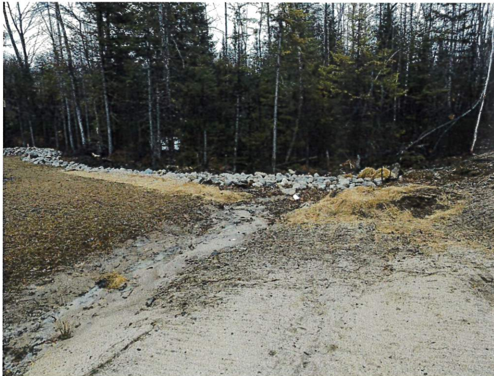
Photo #4 – Reconstructed Level Spreader at Entrance to Buffer #1; Lot 3 Requires Erosion Control Above Swale
