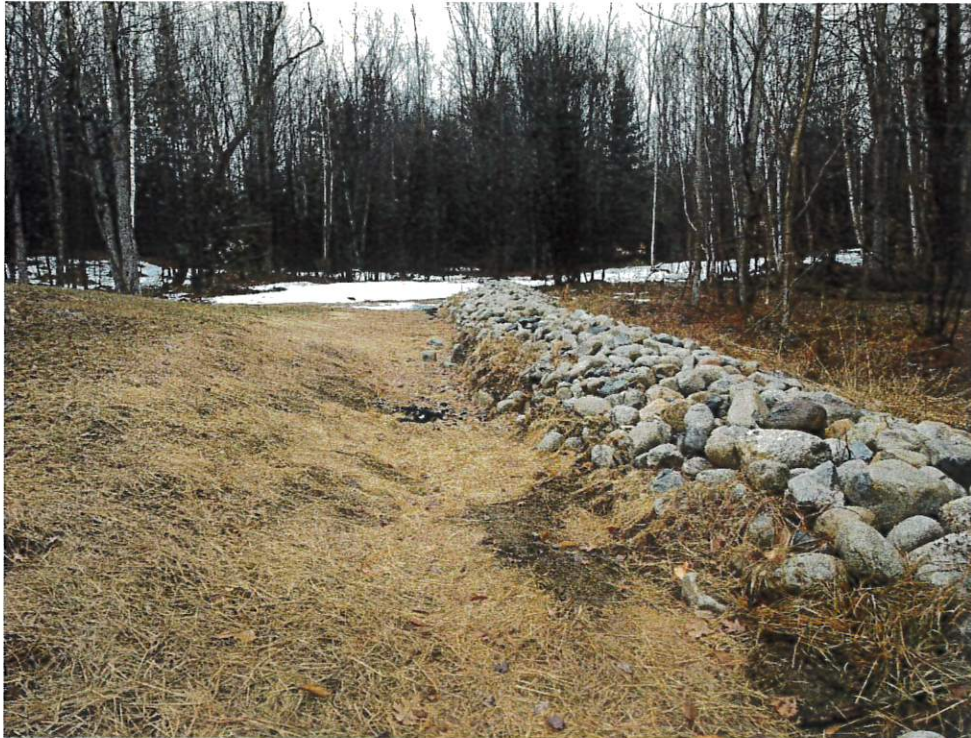
Photo #1 – Level Spreader at Stormwater Buffer 2
