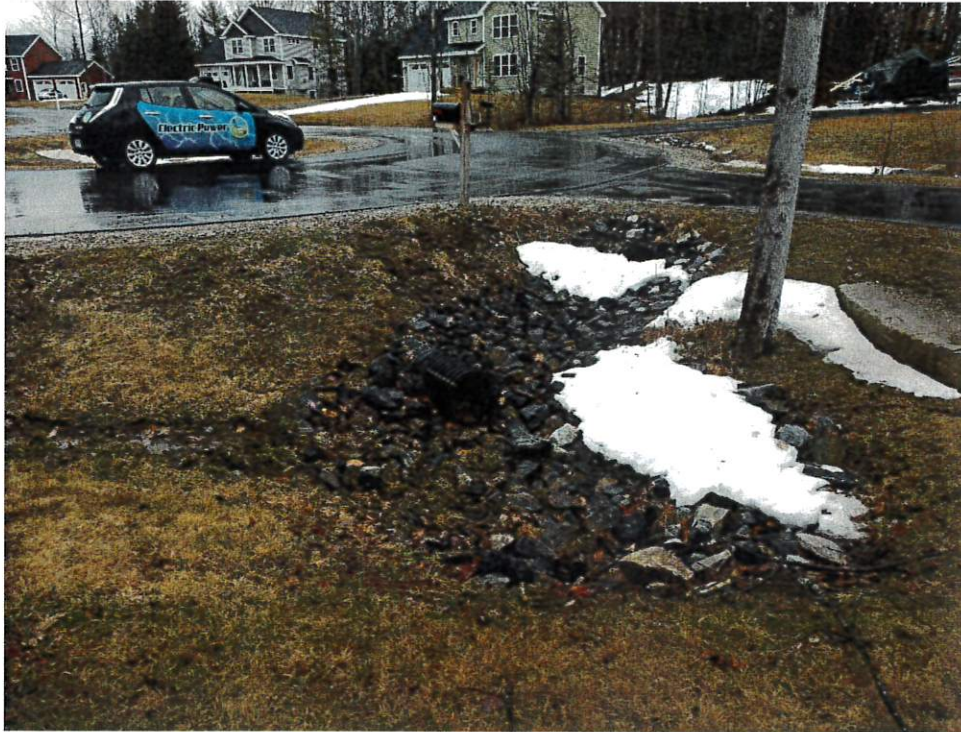
Photo #3 – Culvert from Cul-de-Sac to Stormwater Buffer 2
