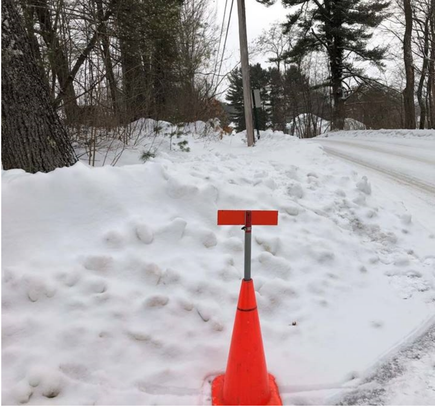
Cone roughly at location where sight distance would be measured at proposed road. Snowbank blocks ability to measure sight distance accurately
