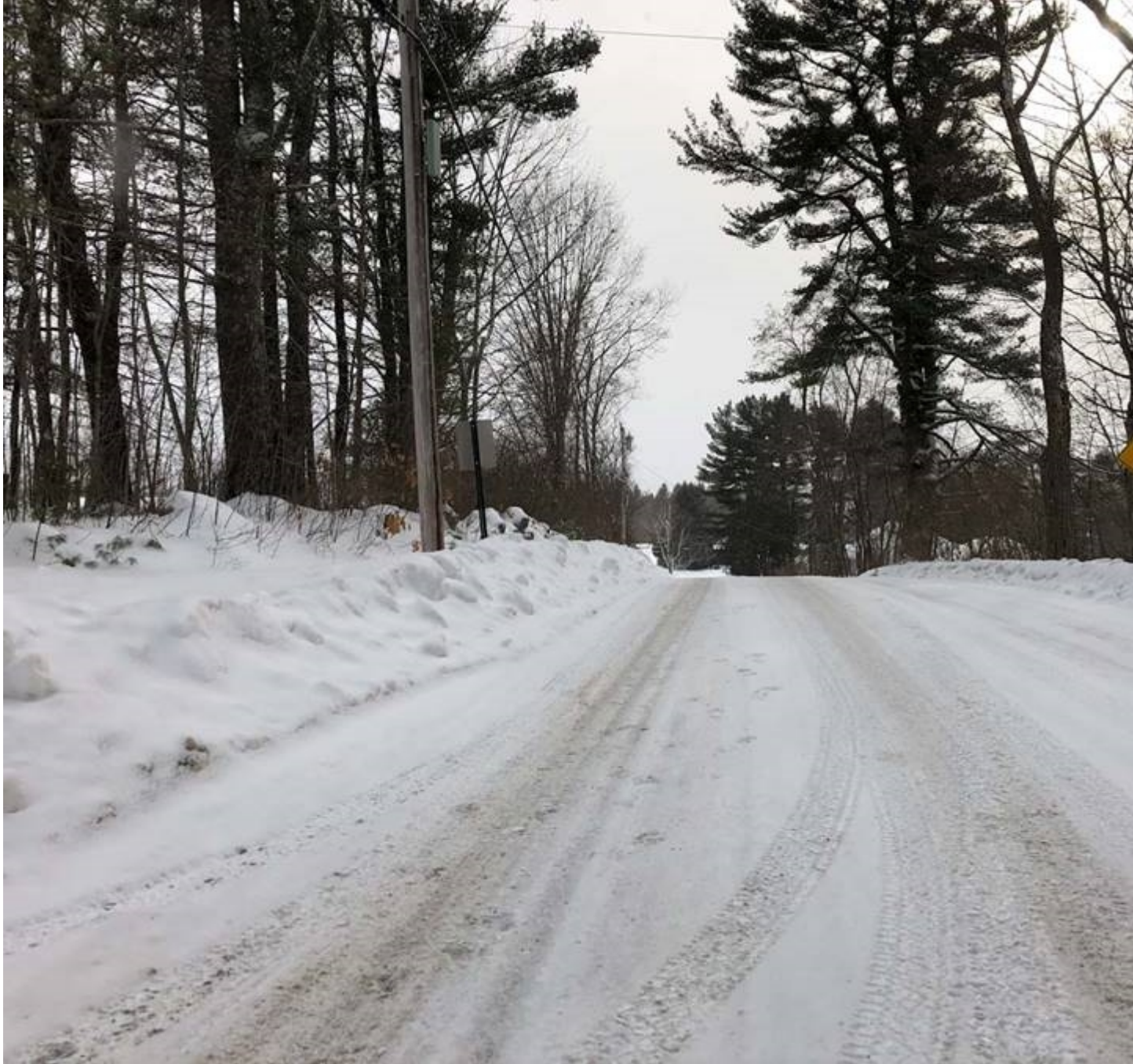
Looking back towards Windham Center Road at edge of traveled way on Nash Road approximately straight out from where sight distance would be measured
