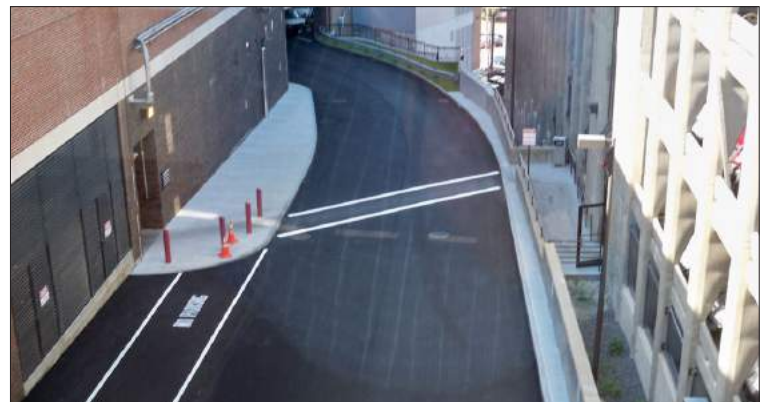
Grade changes and existing infrastructure created opportunities for creative solutions
