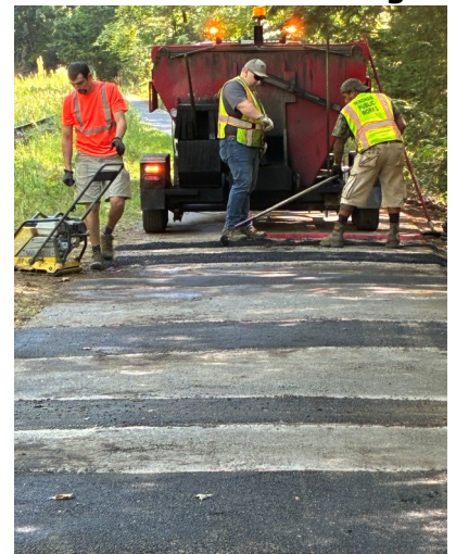
Mountain Division Trail Repair
