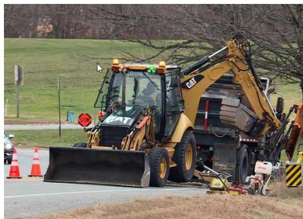
Route 202 Emergency Sinkhole Repair
