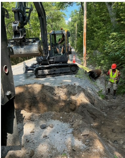
Nash Road Cross Culverts
