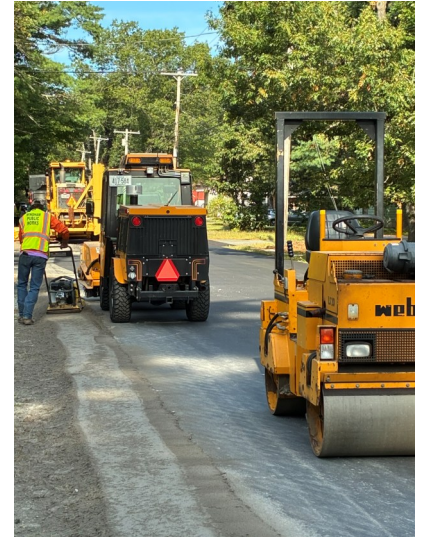
Falmouth Road Paving
