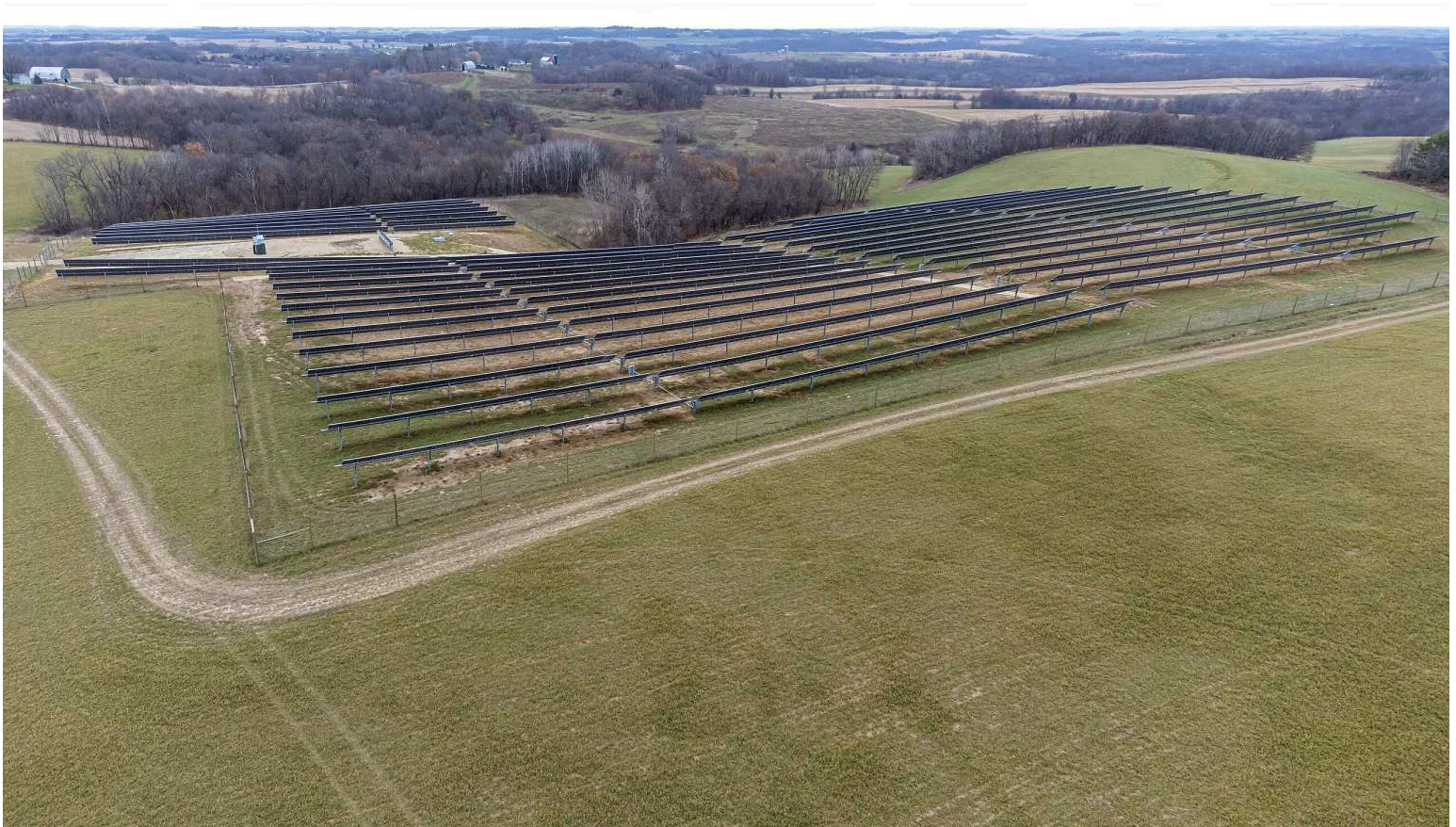
A solar farm near Wheatland, Wisconsin. Credit: Wikimedia Commons
