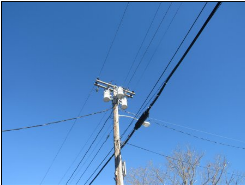
Three pole-mounted transformers located on the eastern portion of the Site.
