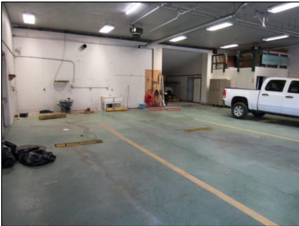
View of the floor trenches in the garage bays.
