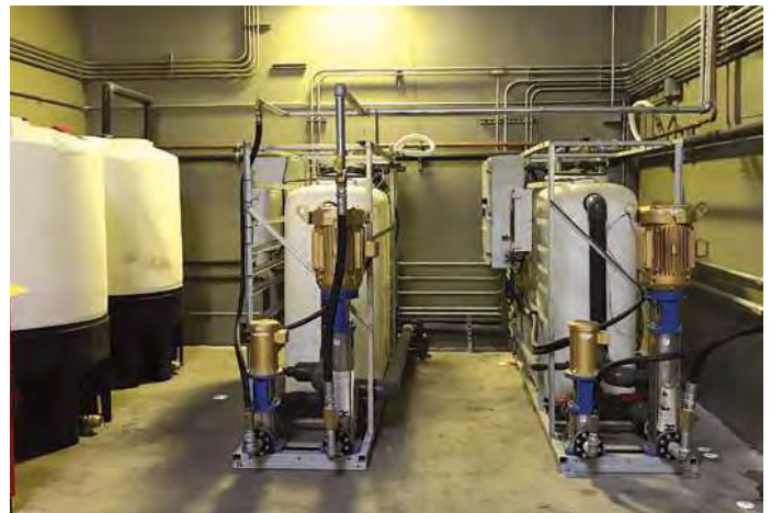
Dual Reclaim water recycling systems at MARTA Perry
