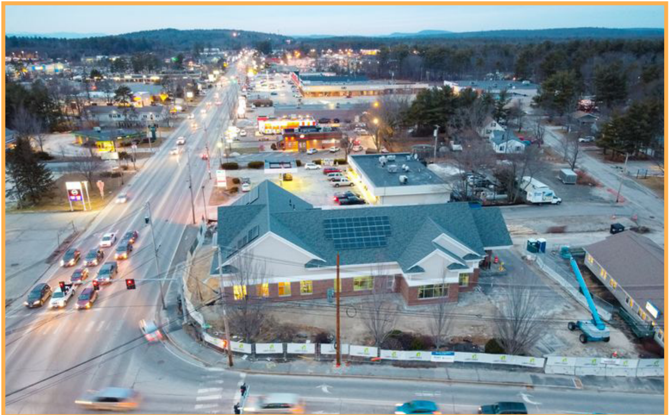
Aerial of North Windham and Bangor Savings Bank with Solar (Photo by SKY HIGH MAINE)
