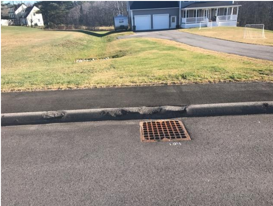
Photo 1 – Recommend adding additional shoulder loam material at the intersection of Chute Road and Georges Lane.
