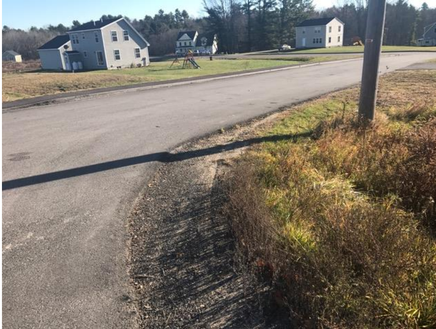
Photo 1 – Recommend adding additional shoulder loam material at the intersection of Chute Road and Georges Lane.
