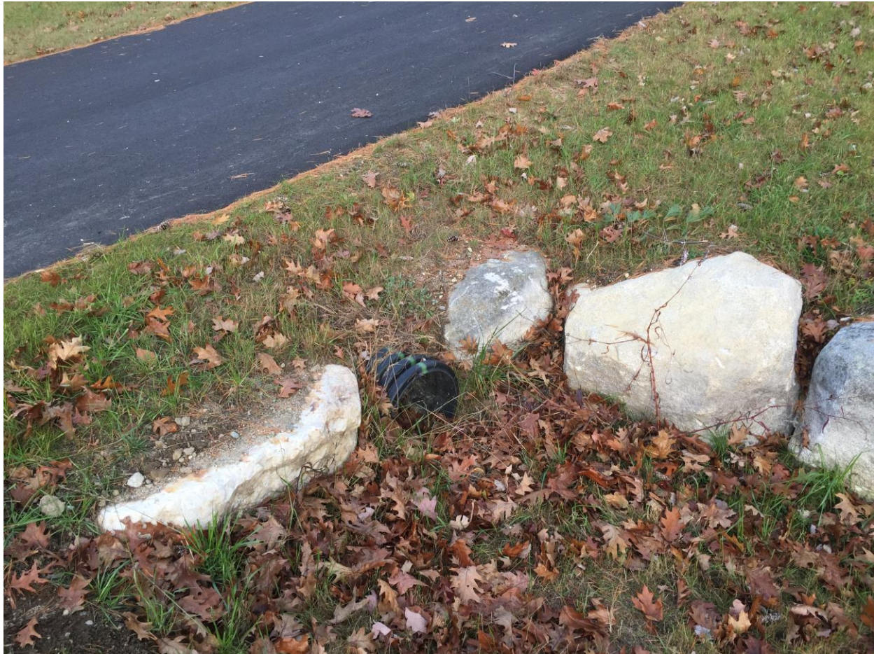
Photo 1 - Construct Riprap Aprons (#79 Harvest Hill Rd).
