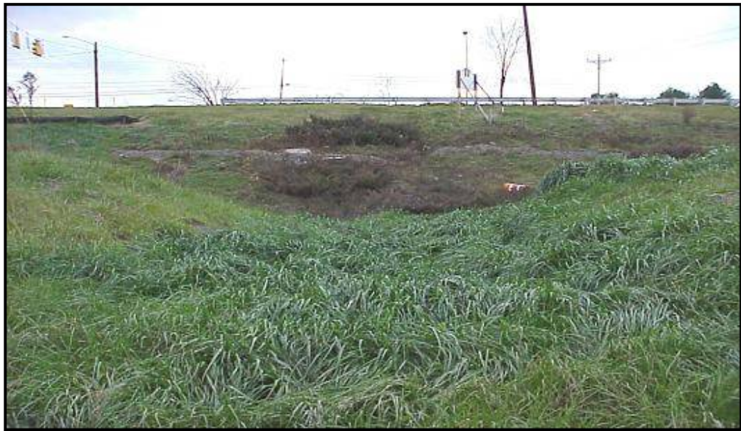
VEGETATED SWALE UNDER CONSTRUCTION WITH HAY BALE CHECK DAM TO REDUCE VELOCITIES
