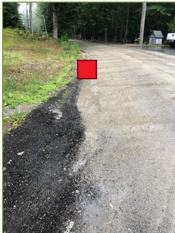
Figure 11. Proposed location of NDS 24-inch deep catch basin on west side of Lakeside Drive at Site 5-5.
