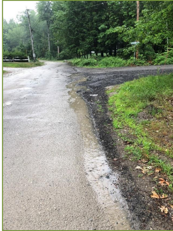
Figure 6. Channelized runoff flowing south along the eastern side of Lakeside Drive toward the James Way intersection at Site 5-5.
