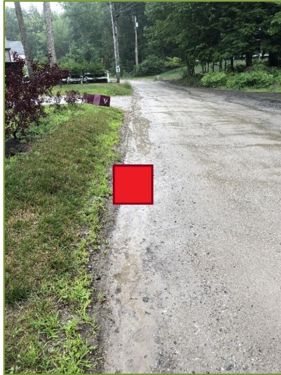
Figure 10. Proposed location of NDS 24-inch deep catch basin on east side of Lakeside Drive at Site 5-5.
