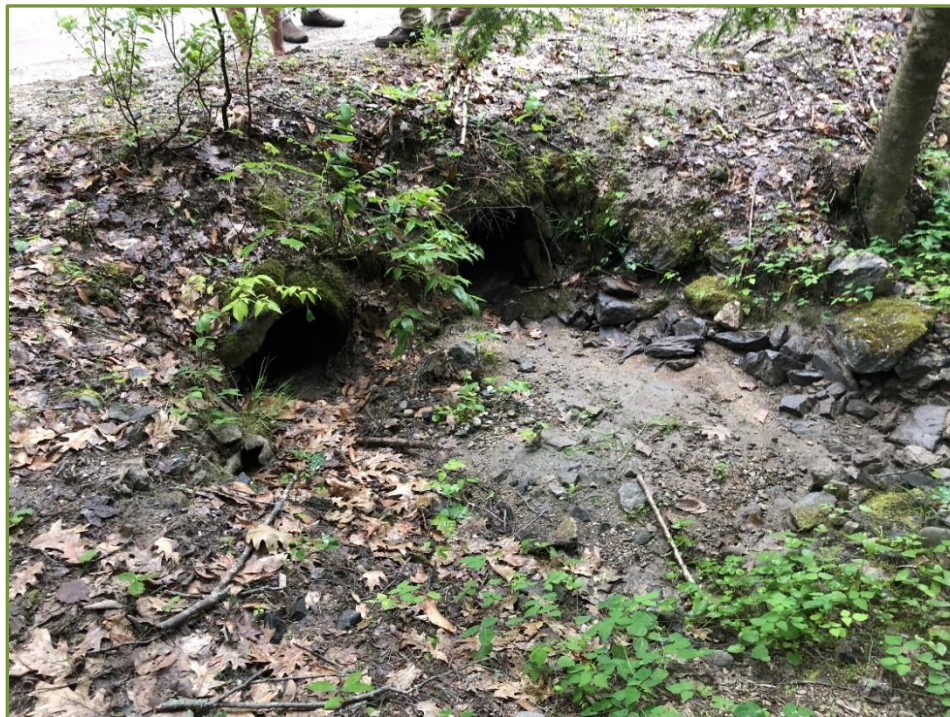
Figure 14. Sediment deposit in the downstream plunge pool at Site 5-11.
