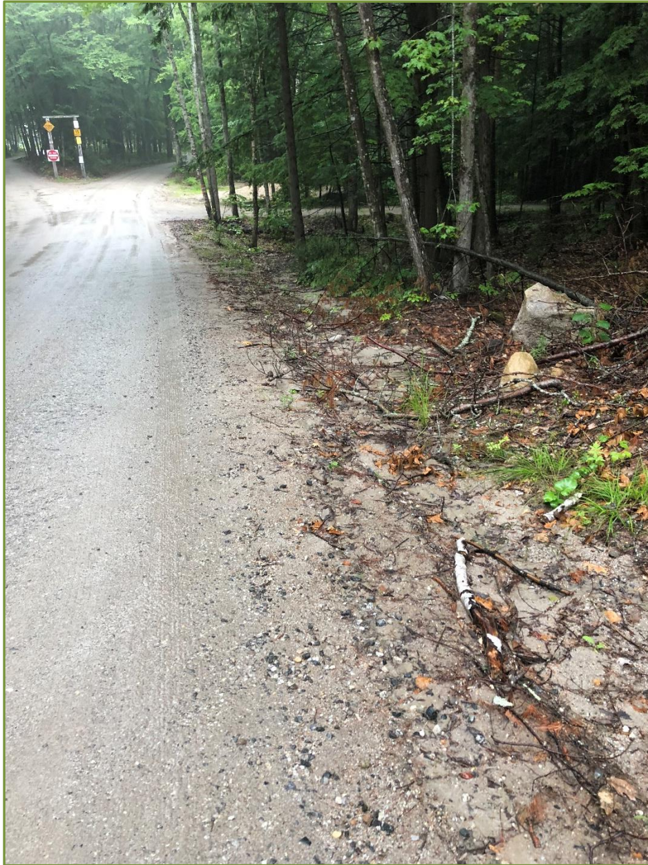
Figure 15. Sediment is being transported along the eastern side of Lakeside Drive as the road approaches Site 5-11.
