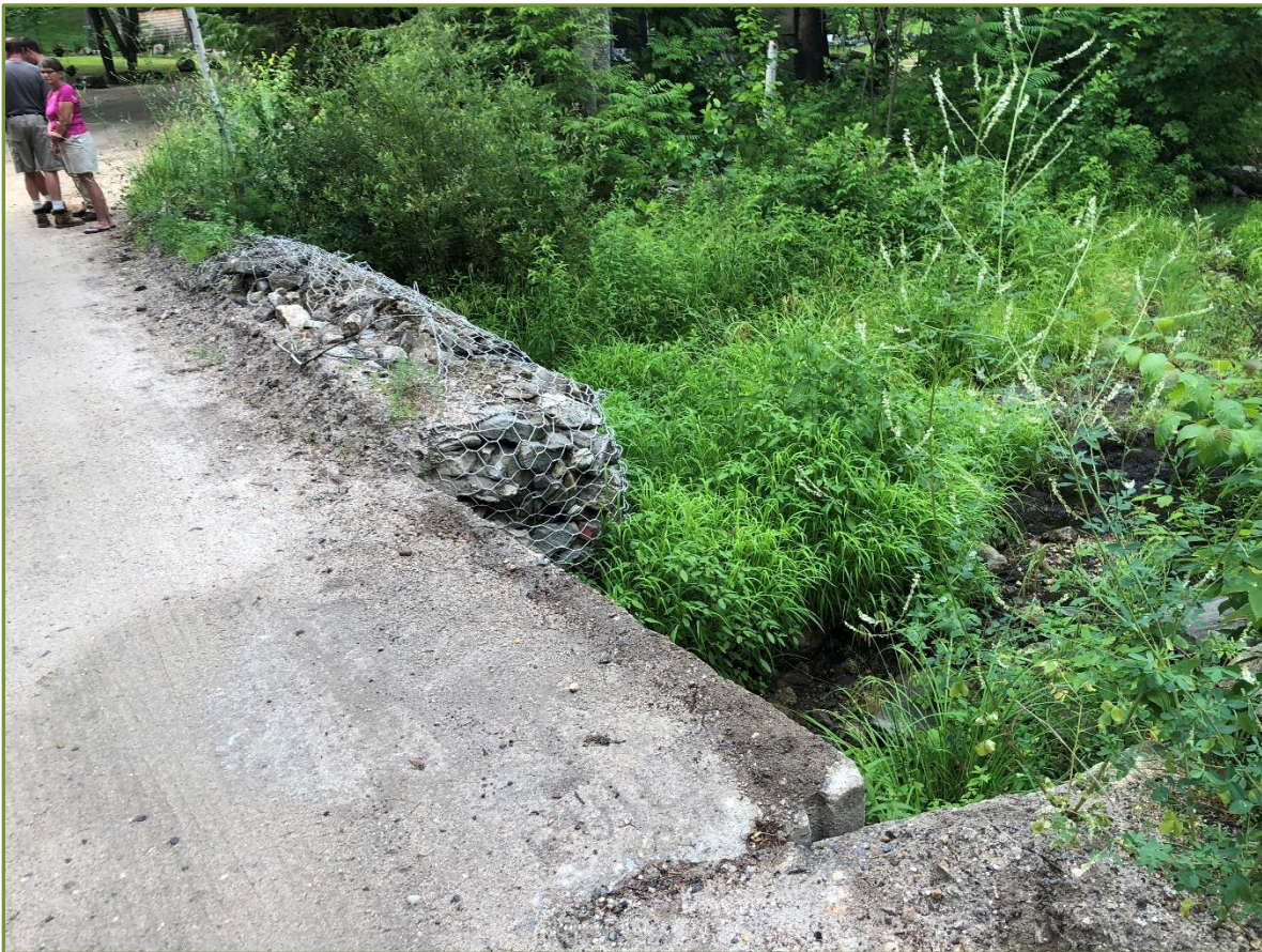
Figure 5. Gabion baskets at Site 5-2 are open, filled with sediment, and have vegetation growing.
