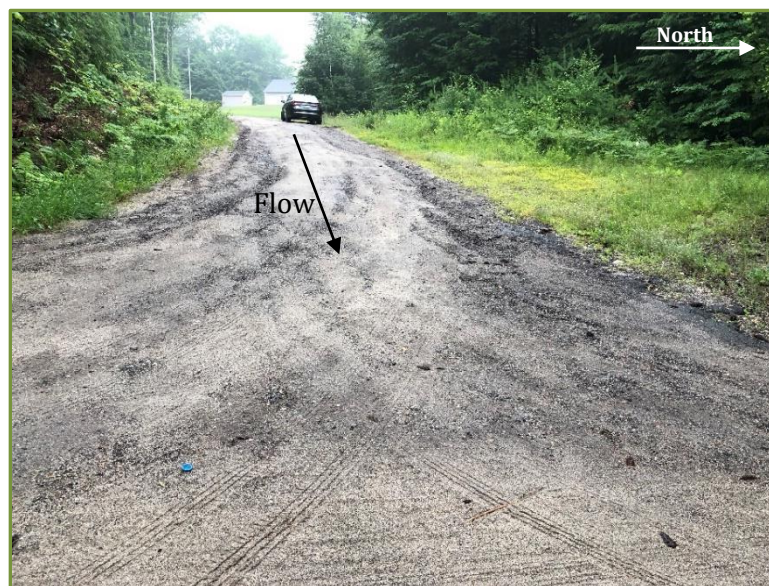
Figure 2. Evidence of channelized runoff coming off Cypress Hill Drive at Site 5-1 (facing west).
