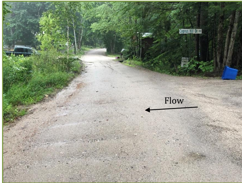
Figure 3. Evidence of channelized flow on Lakeside Drive (left to right) from Cypress Hill Drive, at Site 5-1 (facing south).
