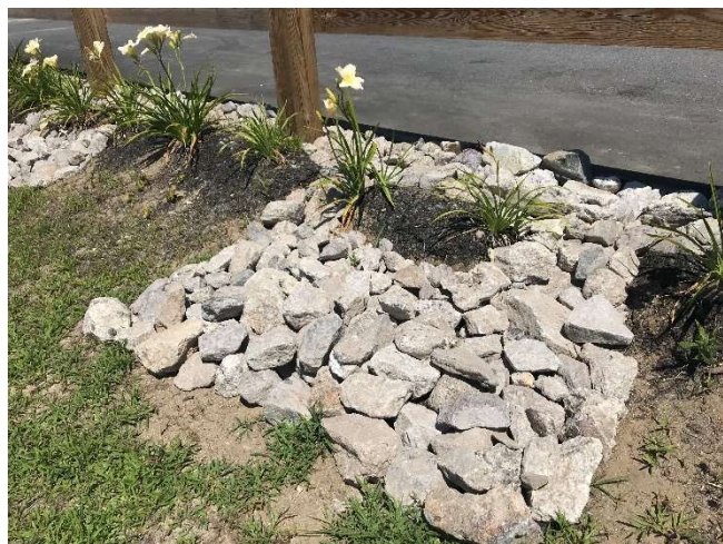
P4: Riprap lined downspout to infiltration basin
