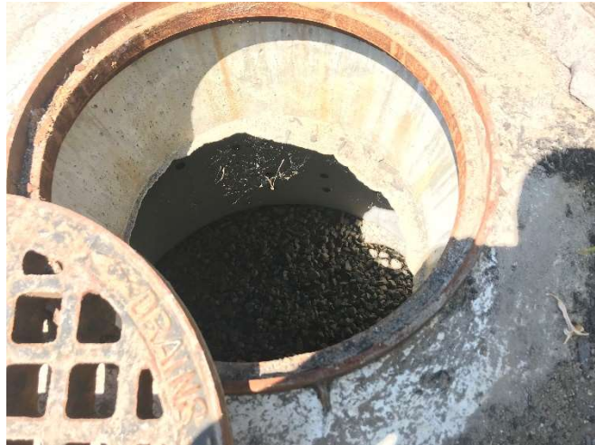
P2: Measuring sediment levels in dry well
