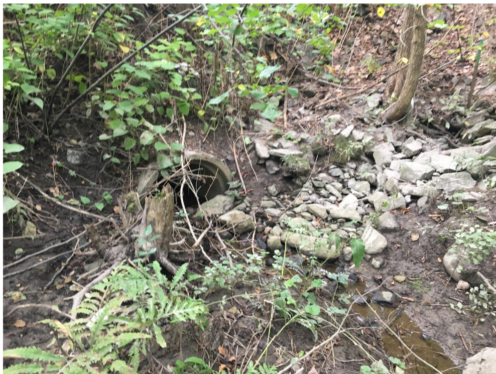
Photo 5: View of culvert inlet to the south of the site that drains Wetland A1 under Depot Street.
